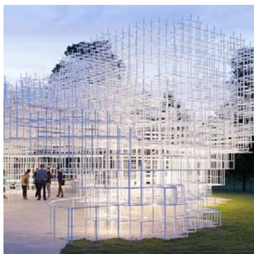
Sou Fujimoto, Cloud - Serpentine Pavilion Structure. Stainless Steel + Glass. 2014 — Cube frames form a visual description of discipline, precision and order. From the interior a feeling of nested comfort is perforated with glimpses of external sounds + sights.
